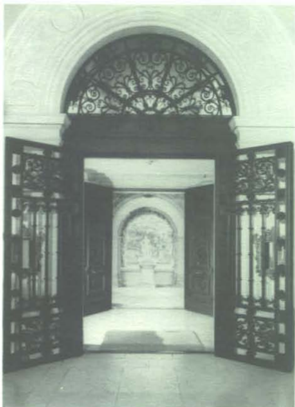
The entrance doors of The Breakers , looking northwest. H.A.B.S. photo by Jack E. Boucher, 1971. RIHS Collection (RHi X3 6198).
