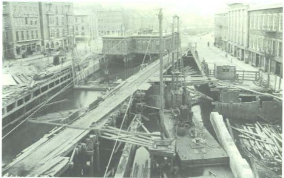
Providence carried out a vigorous bridge-building program between 1892 and 1897. This photograph, taken by an unidentified photographer in 1893, shows the reconstruction of the retaining walls along the Providence River at its convergence with the Woonasquatucket and Moshassuck rivers. RIHS Collection (RIHS X3 6994).
